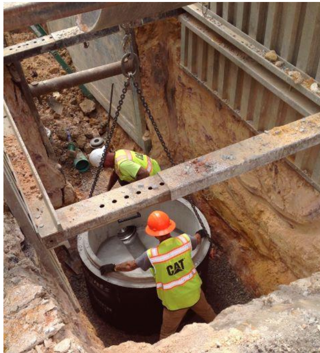
Photo 4: Wet-well installation
