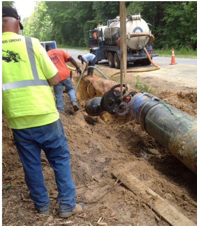
Photo 3: Preparing for installing line using bore.
