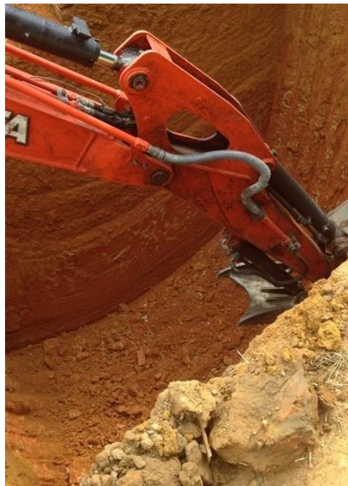
Photo 2: Trenching for line
