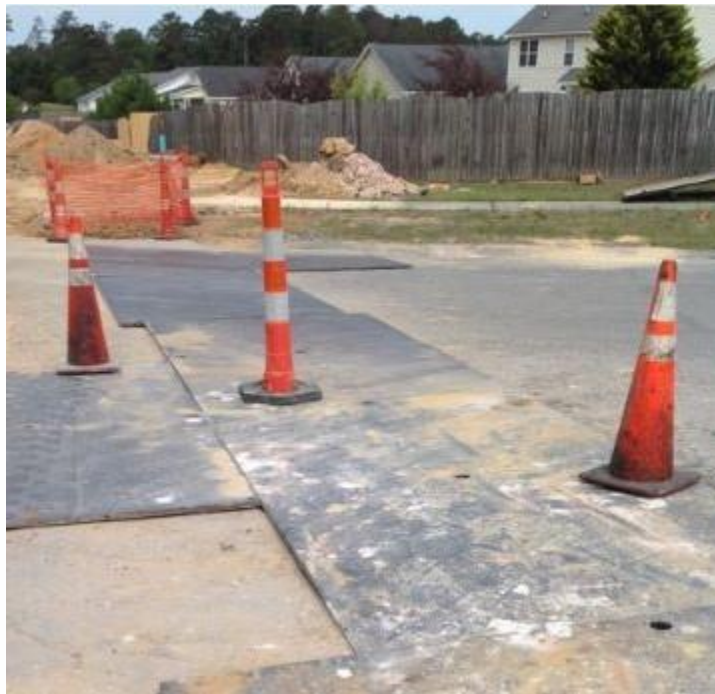
Photo 5: Gravity Line Crossing Bitternut Road
