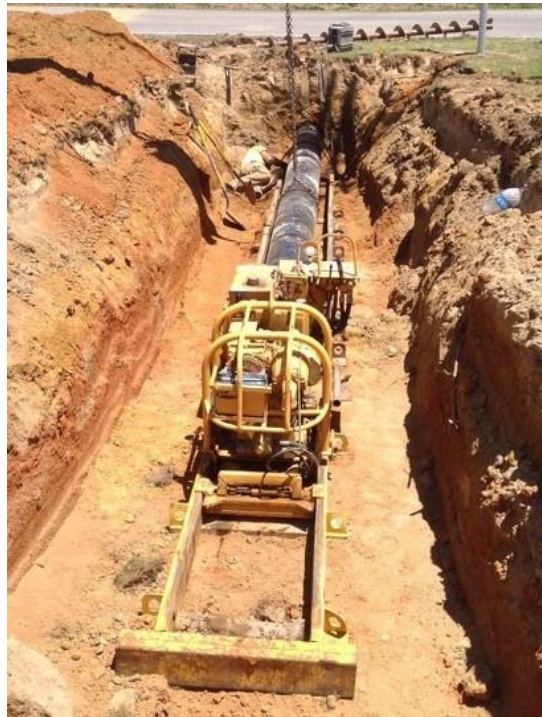
Photo 3: Installing line using bore and jack.
