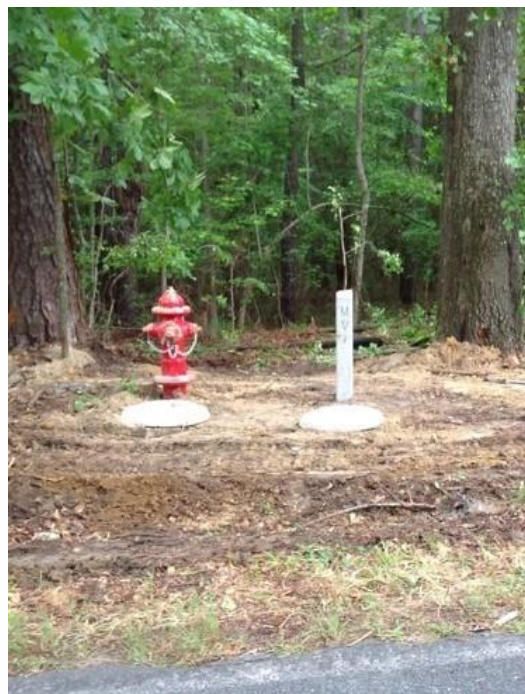
Photo 2: Fire hydrant install
