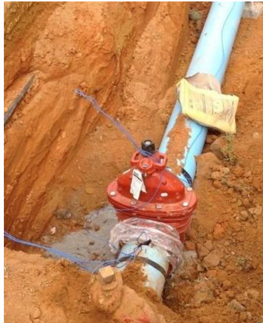
Photo 1: Valve Install
