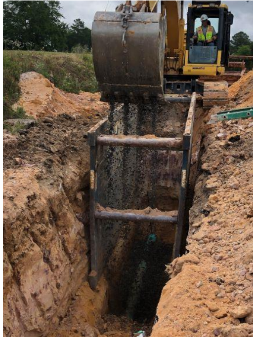
Photo 1: Laying line on Lower Richland Boulevard
