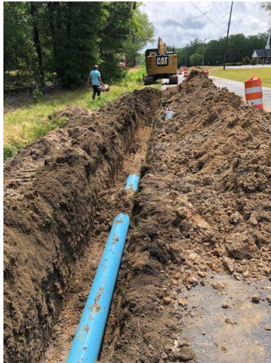
Photo 4: Line installed Cabin Creek Road
