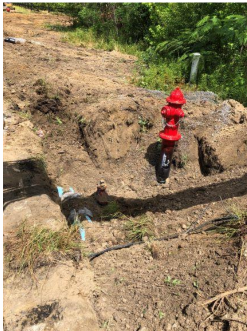
Photo 2: Fire hydrant install
