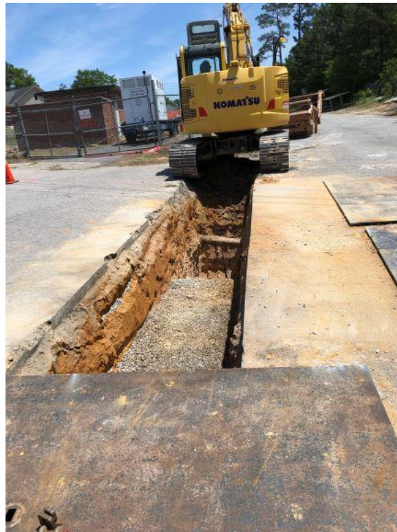
Photo 5: Line install Bitternut Drive
