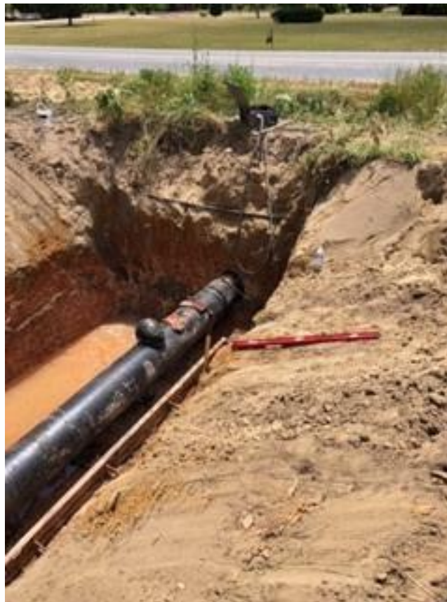
Photo 3: Installing line using bore and jack.
