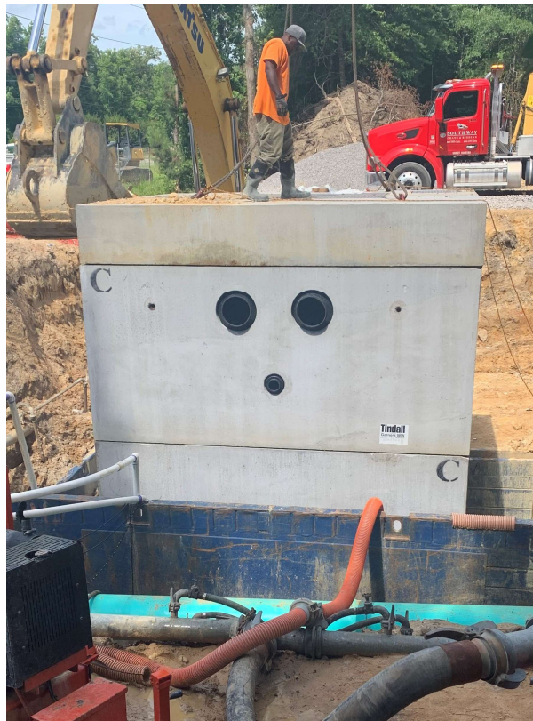
Photo 1: Wet-well install
