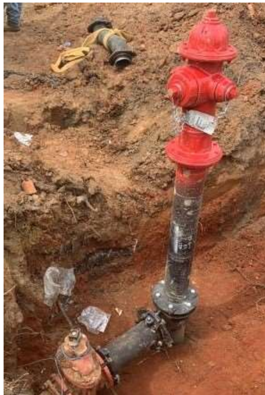
Photo 2: Fire Hydrant install
