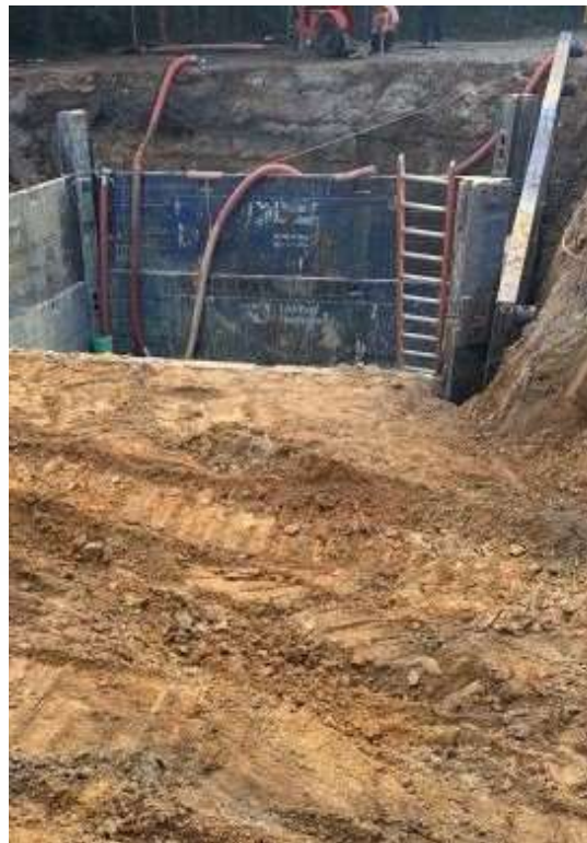
Photo 1: Wet-well install
