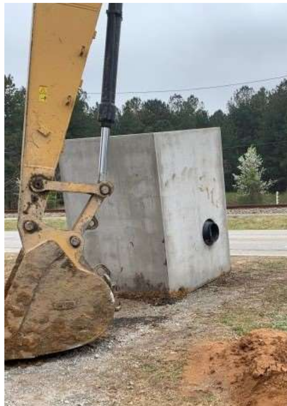
Photo 2: valve box install
