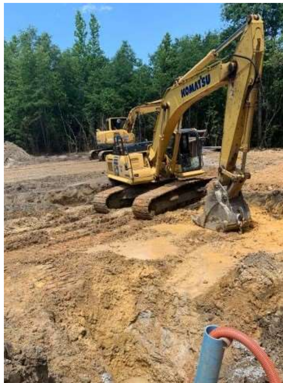
Photo 1: Pump Station install
