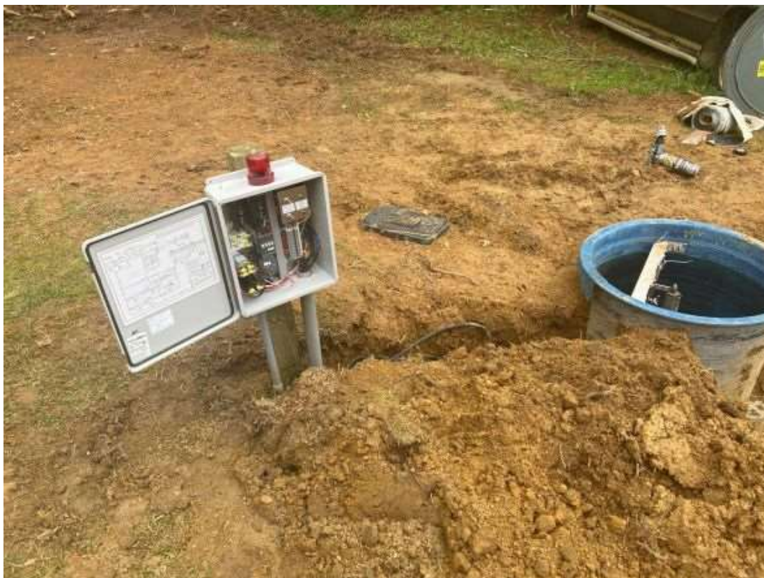
Photo 3: Grinder system install
