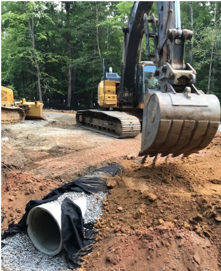
Dirt Road Paving Package M - Tall Oaks Rd
