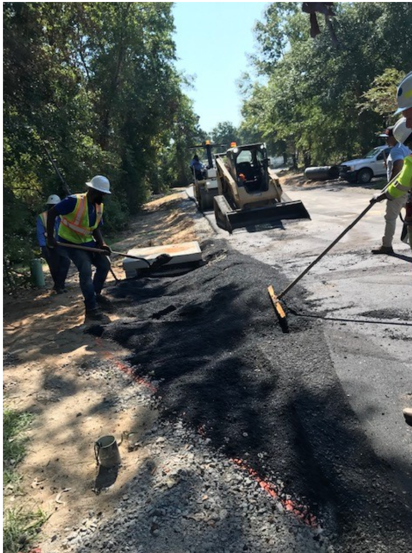
Dirt Road Paving Package M - Bow String Rd.
