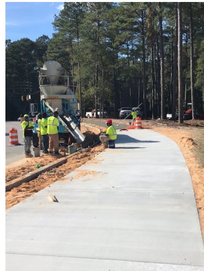
Polo Rd. Curb Installation
