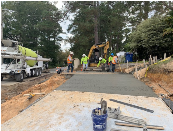
Harrison Rd. Sidewalk Installation
