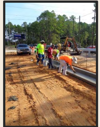
Curb and gutter installation - Clemson Road Widening.
