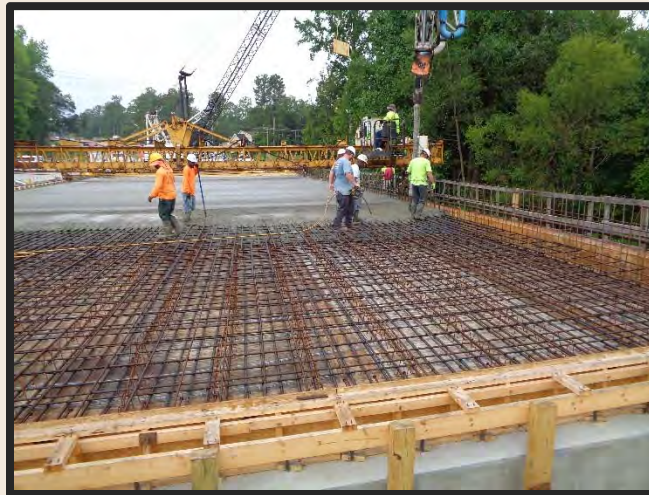
Concrete bridge pour – Hardscrabble Road Widening.
