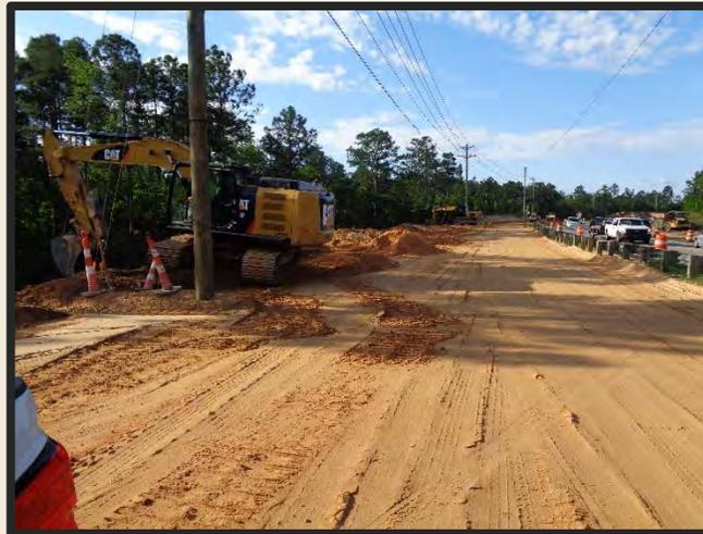
*The Clemson Road Widening Project takes shape with clearing and grubbing, erosion control measures, earthwork, and drainage installation activities underway.*
