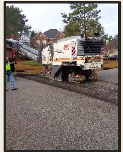
*Milling operations in preparation for resurfacing.*
