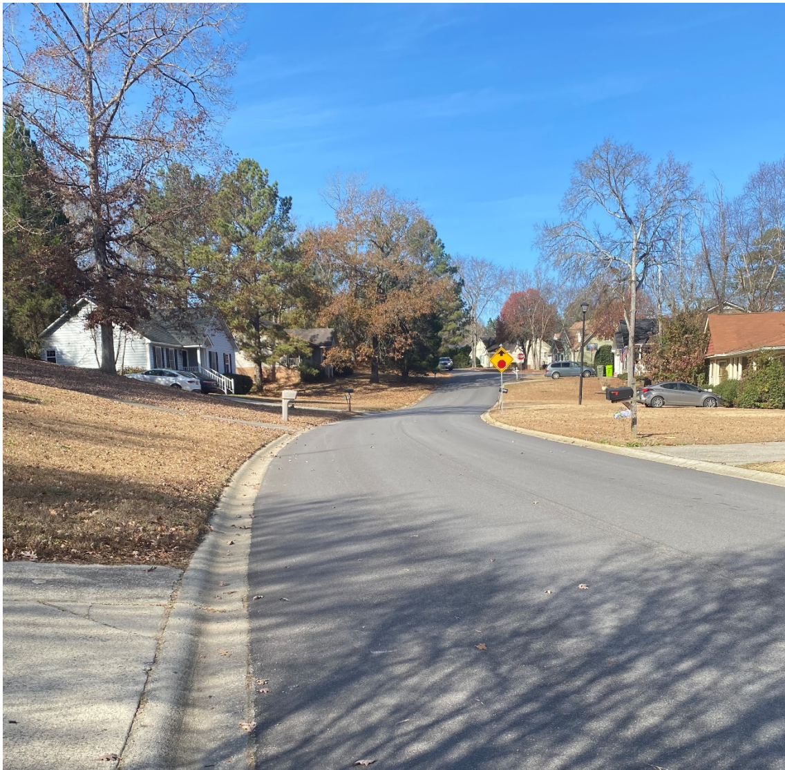
Resurfacing project on Riverwalk Way
