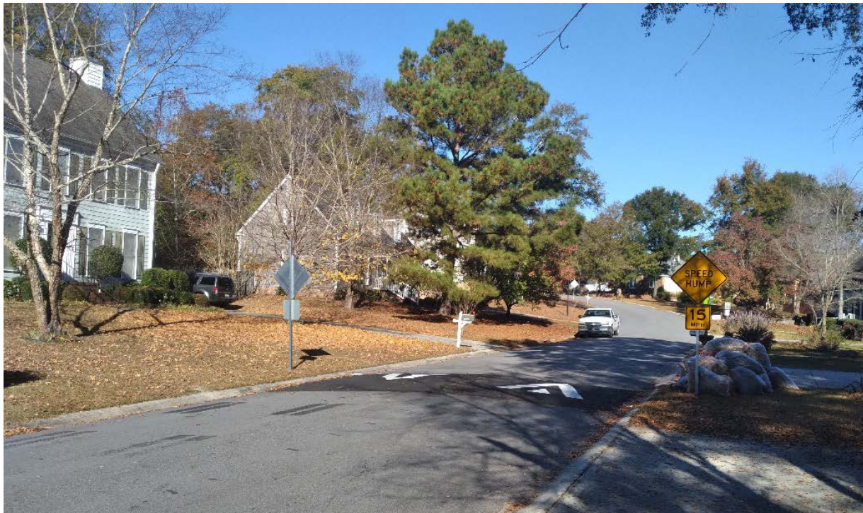
Speed hump installed by RDM on Whitehurst Way
