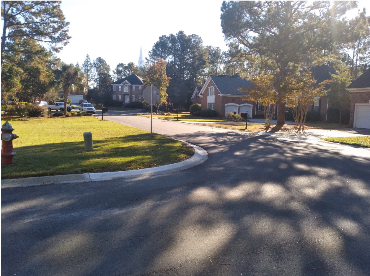
CIP resurfacing project on Hollingwood Dr
