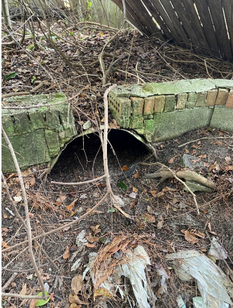
Clogged outfall pipe (before)
