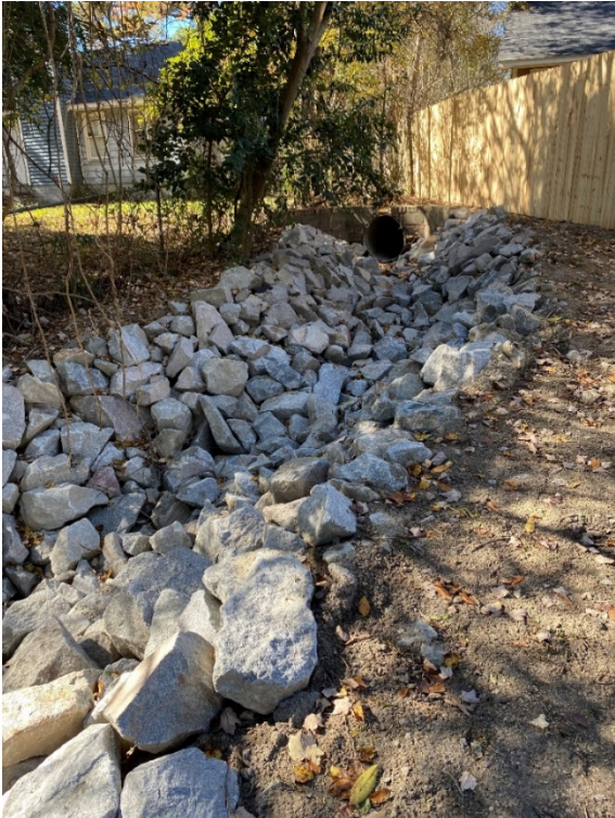
Clogged outfall pipe (before)
