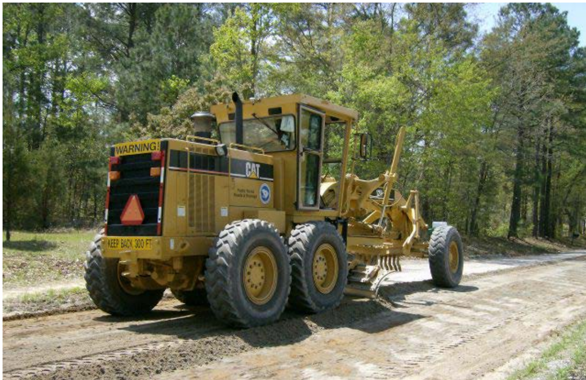
Unpaved road scrape performed by RDM crew
