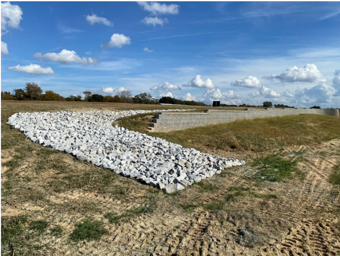
Drainage improvement project at CUB
