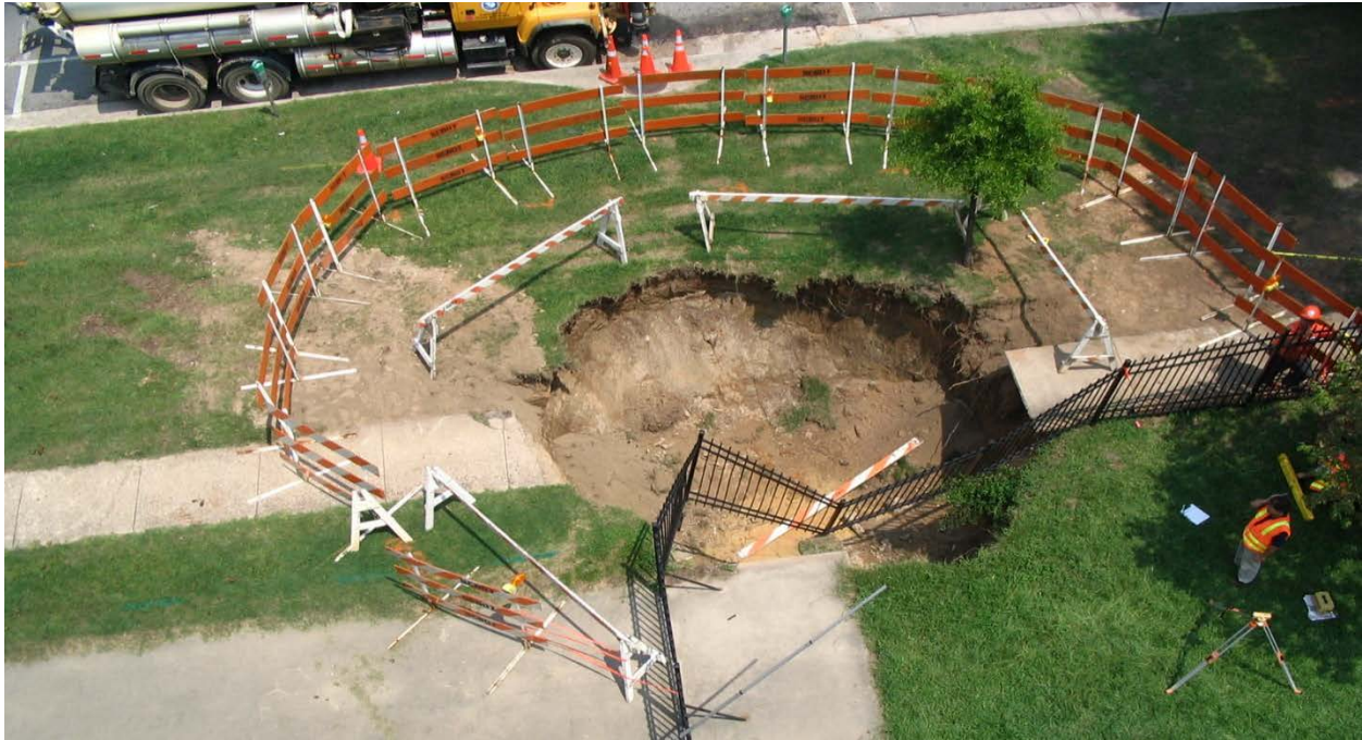
Sinkhole near 2020 Hampton St
