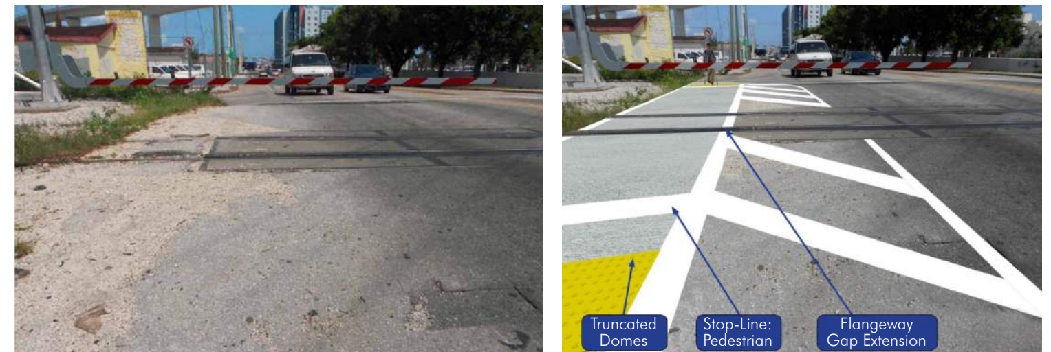
Figure 41: Before and after bike/pedestrian railroad crossing
