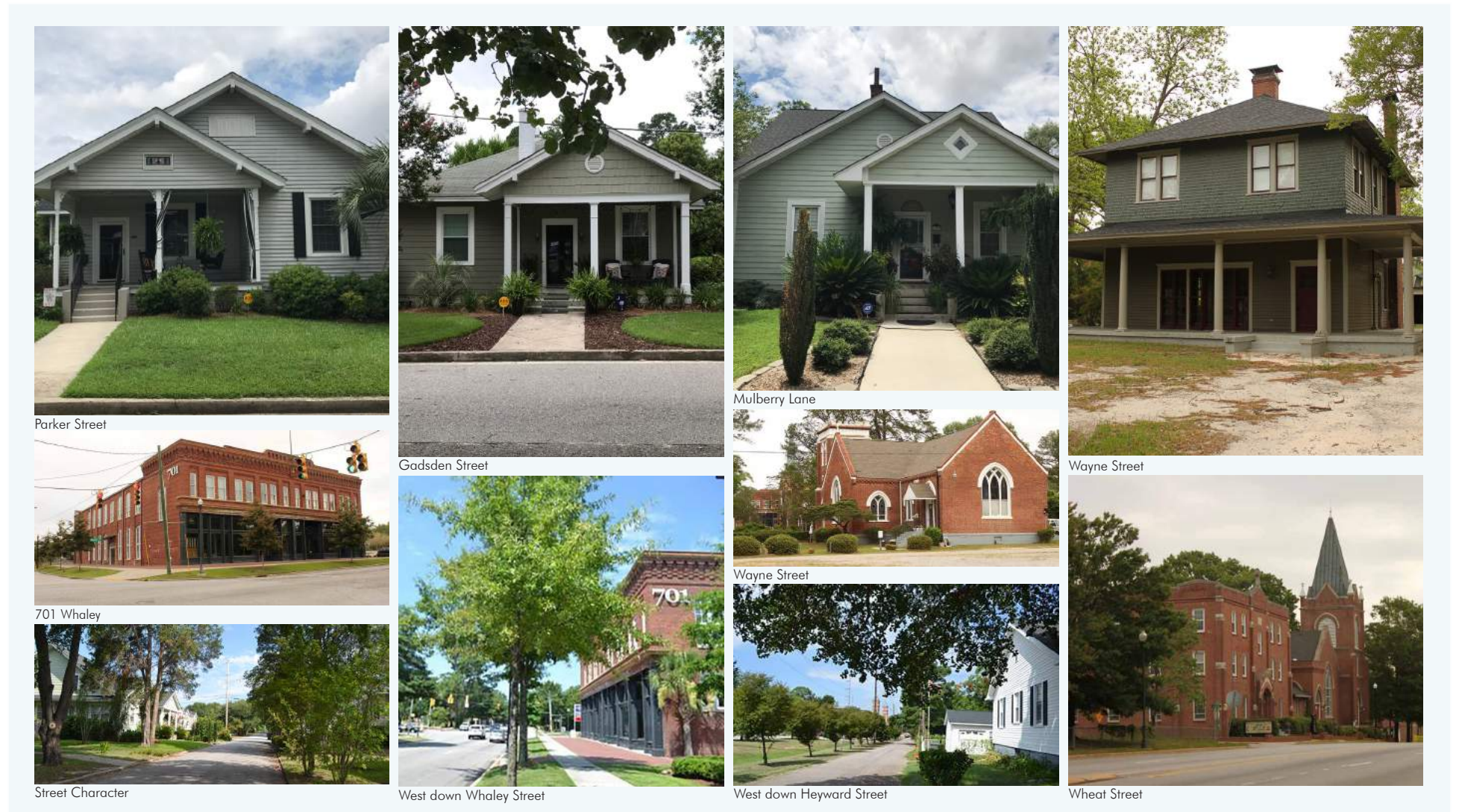
Figure 6: Existing Architectural Inventory - Whaley Neighborhood sub area
