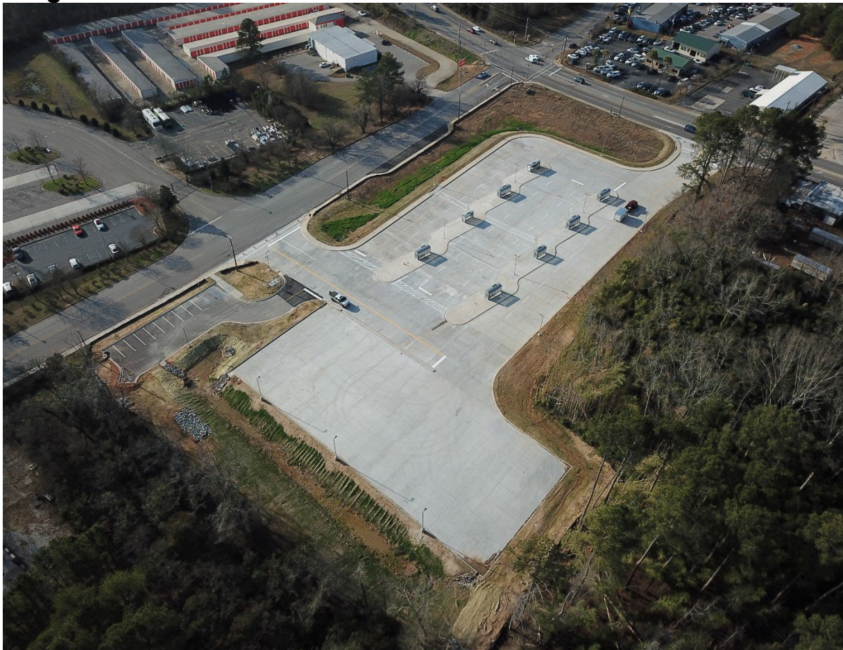
Aerial view of the Lucius Road Superstop Project.
