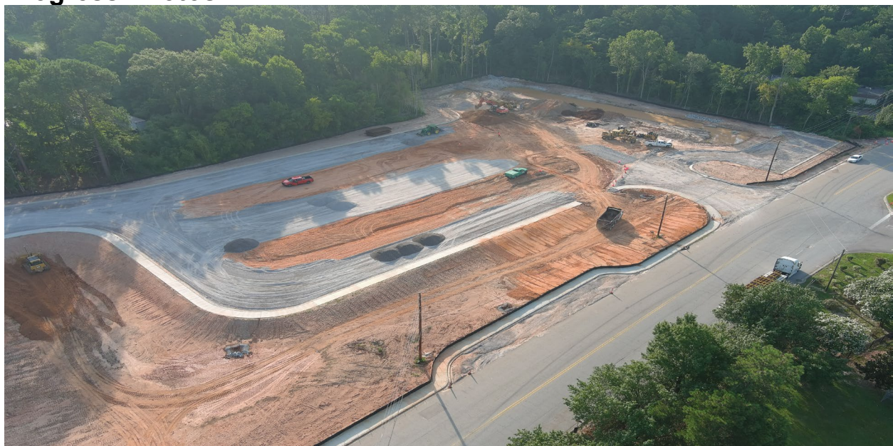
Aerial view of the Lucius Road Superstop Project.
