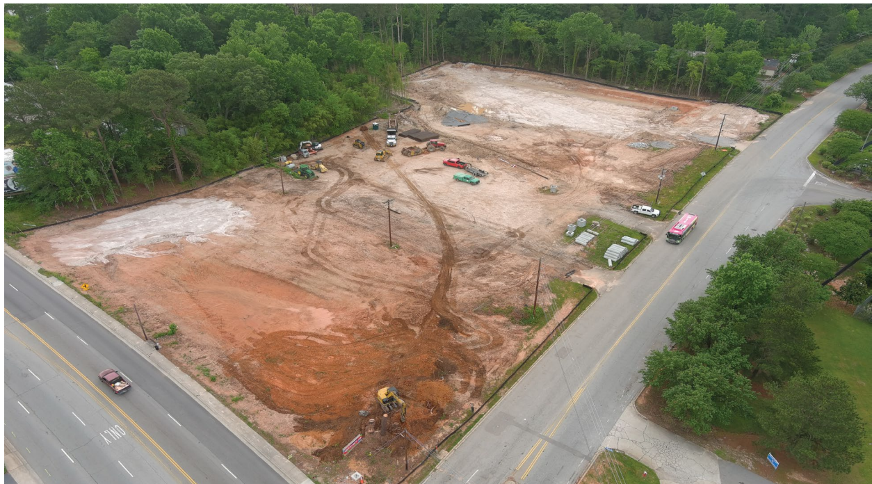
Aerial view of the entire Lucius Road Superstop Project.
