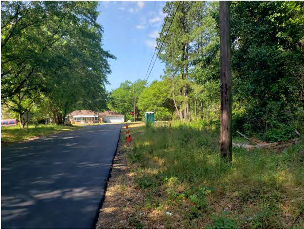
Southern portion of site.
