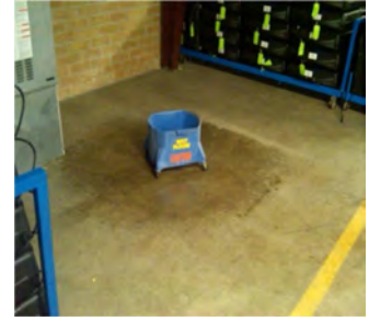
Elections & Voter Registration Warehouse Water Leak
