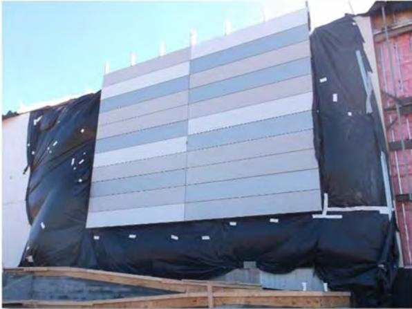
New insulated metal panels at exterior
