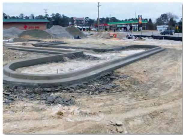
New curb and gutter installation at front lot
