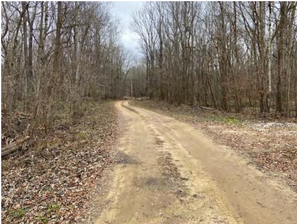
Existing Dirt Road Access to Bridge with Typical Wooded Floodplain in Winter
