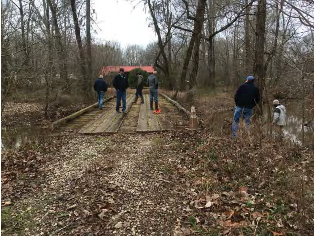
Existing Bridge Crossing – Facing West – Flow Direction from RT to LT
