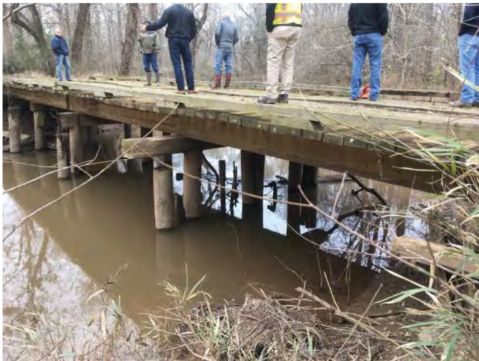
Existing Bridge Crossing Facing Upstream Showing Superstructure and Pile Bents
