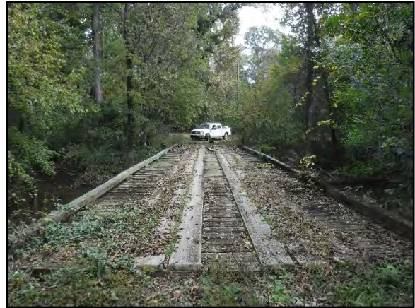
Photo 1 – RCCC Dirt Road Bridge, Richland County, South Carolina.
