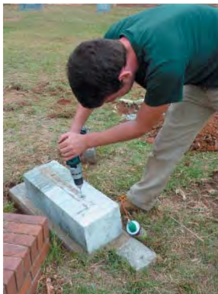
Figure 176: 1014, removing ferrous pins
