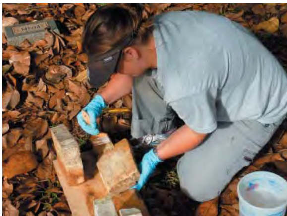
Figure 59: 0514, applying consolidant
