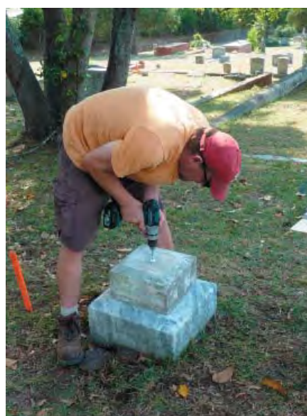
Figure 21: 0490, drilling hole for pin
