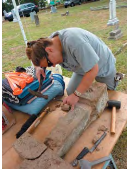
Figure 131: 0980/0981, removing mortar repairs
