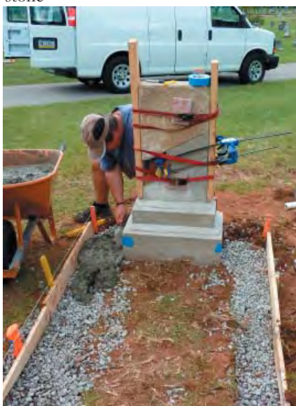
Figure 168: 1013/1016, pouring foundation
