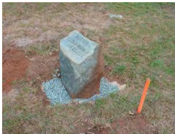
Figure 140: 0986, marker reset
