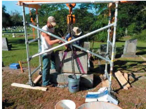
Figure 94: 0644.01, resetting headstone
