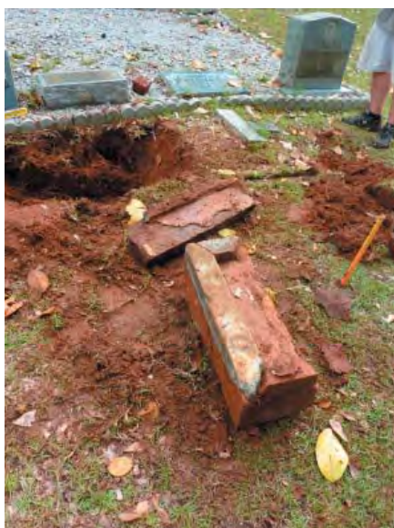
Figure 68: 0537, excavated sub-base and base
