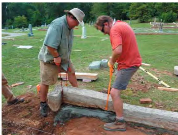
Figure 87: 0565, reinstalling bedstead
