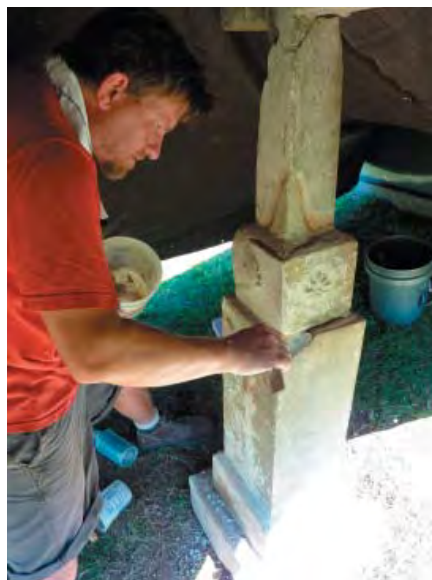
Figure 135: 0980/0981, applying repair mortar
