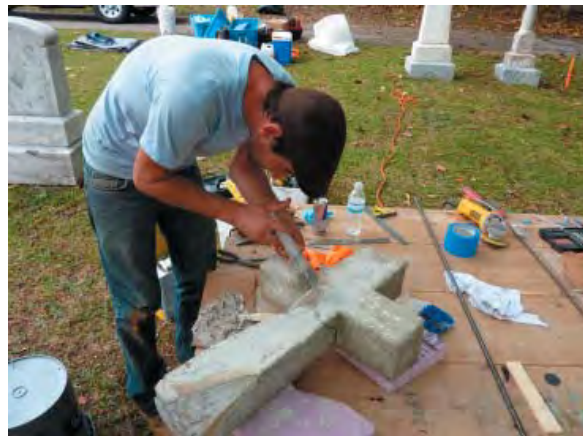
Figure 133: 0980/0981, injecting epoxy
