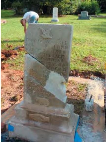
Figure 169: 1013/1016, repair mortar application in process
