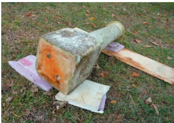
Figure 20: 0490, mortar divets in bottom of pillar
