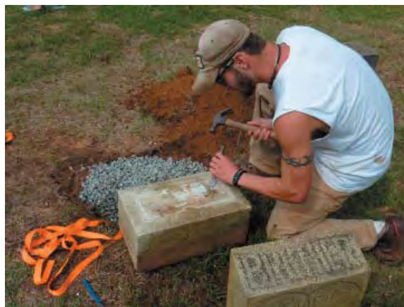
Figure 110: 0913.04, removing mortar
