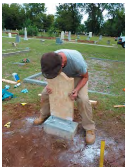
Figure 35: 0501, reattaching tablet
