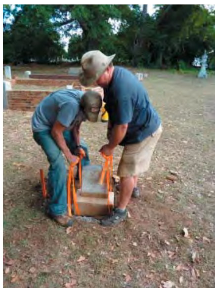
Figure 53: 0511, resetting marker
