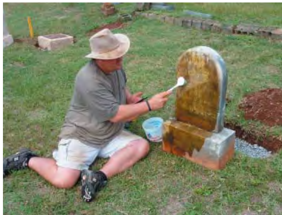
Figure 14: 0470, cleaning marker
