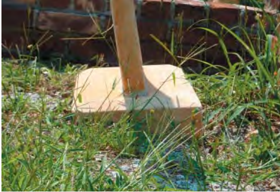
Figure 3: 0001.01, tilted base before treatment
