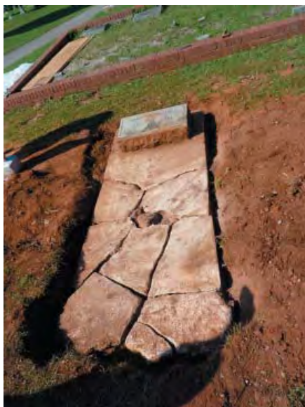
Figure 189: 1015, concrete foundation reassembled
