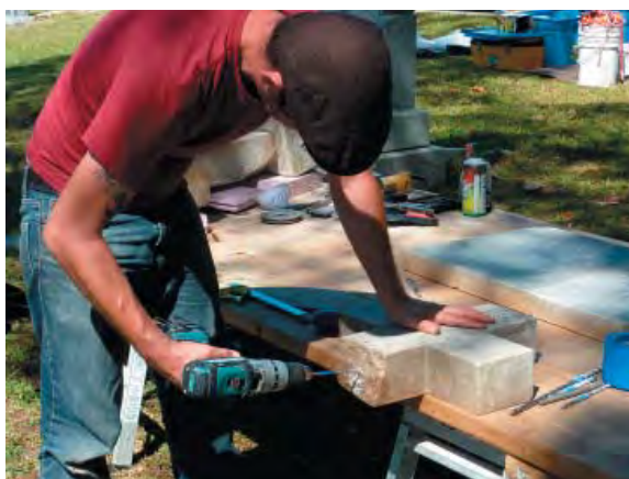
Figure 40: 0505.04, drilling pin hole
