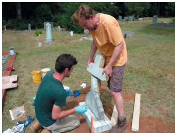
Figure 145: 0990, reassembling marker
