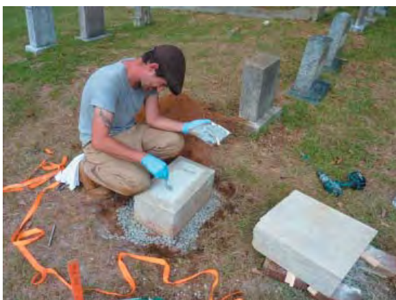
Figure 111: 0913.04, preparing marker for pinning
