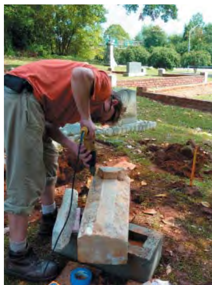
Figure 69: 0537, drilling pin holes
