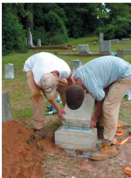
Figure 112: 0913.04, reattaching headstone
