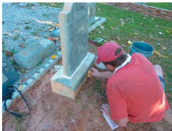
Figure 71: 0537, tinting repair mortar
