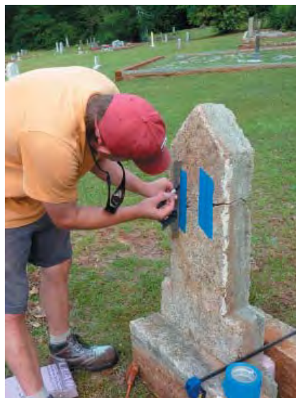
Figure 86: 0565, preparing marker for pinning
