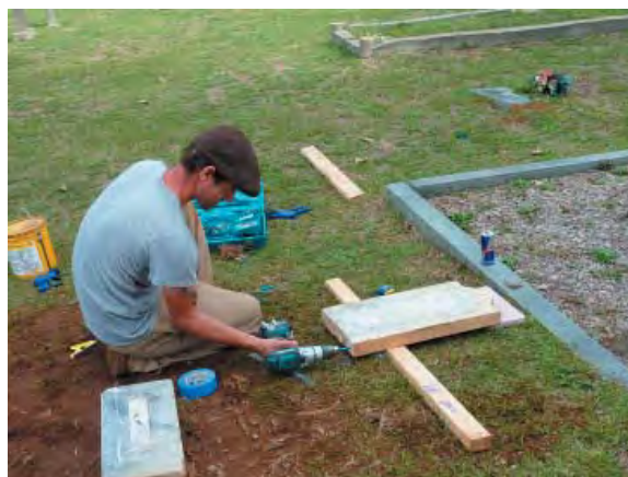
Figure 34: 0501, drilling holes
