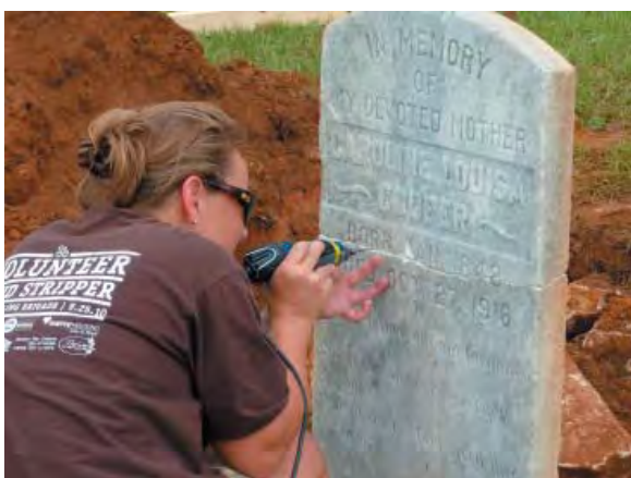
Figure 179: 1014, preparing tablet for repair mortar
