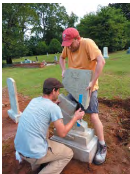
Figure 167: 1013/1016, reassembling headstone
