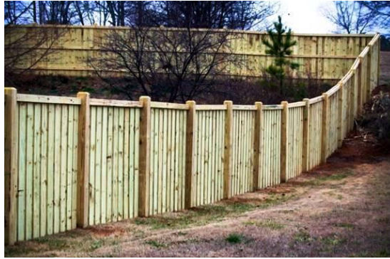
Figure 26-5.8(f)(1): Fence with Finished Side Facing Out
