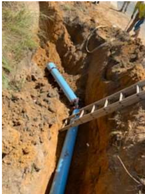
Photo 4: Force main install
