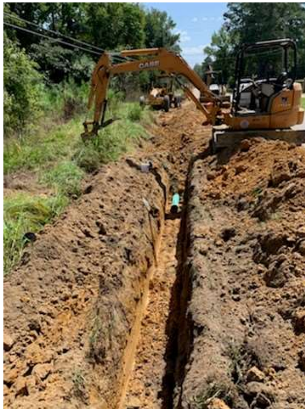
Photo 3: Pipeline installation
