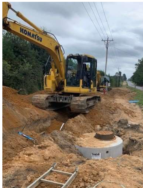
Photo 1: Manhole install
