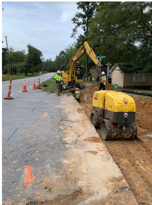
Photo 4: Force main install
