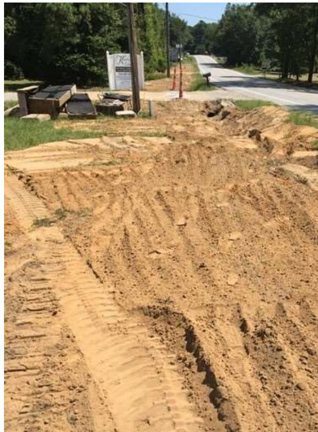
Photo 4: Force main install
