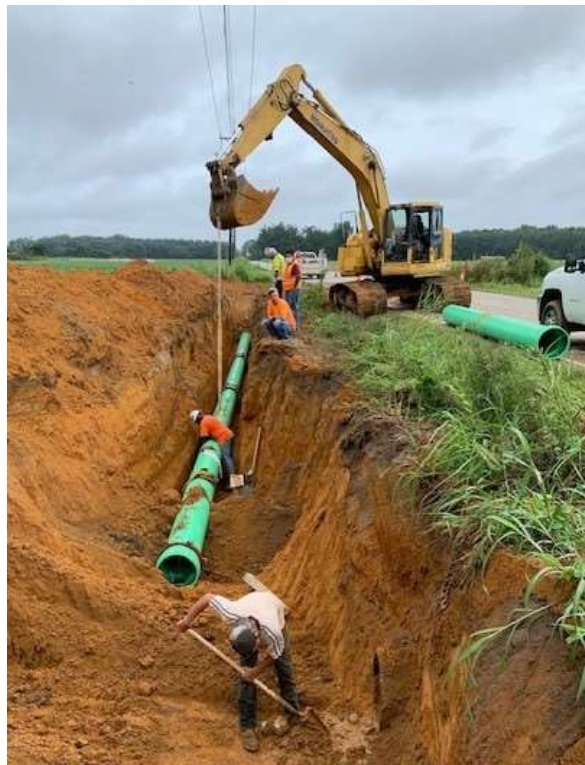
Photo 1: Pipeline installation
