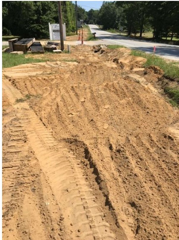
Photo 4: Force main install
