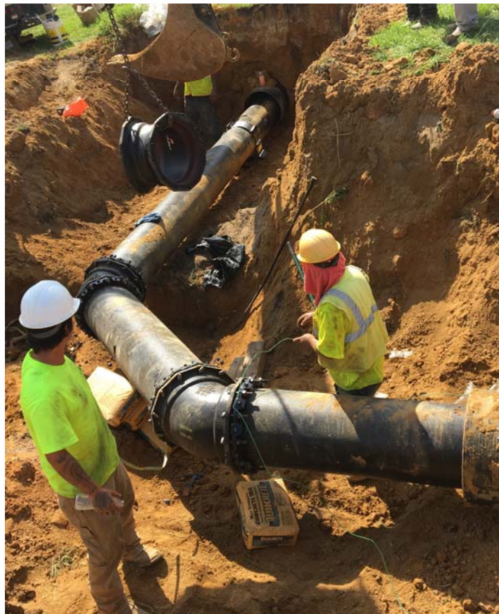
Photo 2: Bore and casing install
