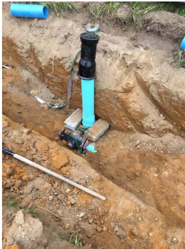
Photo 3: Fire hydrant installation
