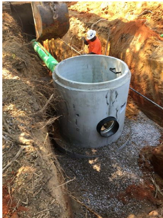
Photo 1: Valve install
