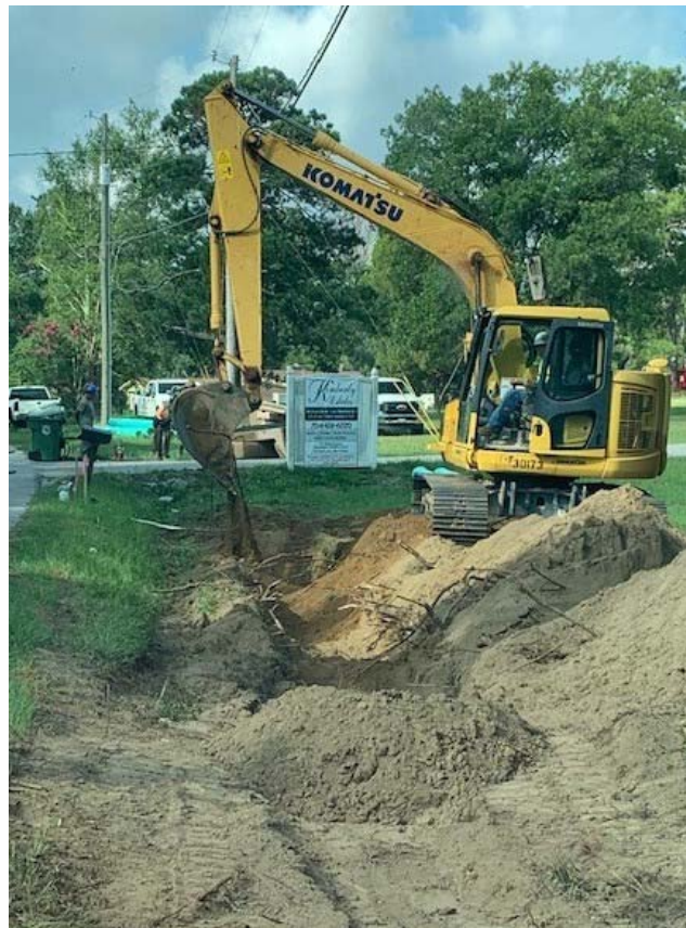
Photo 4: Force main install
