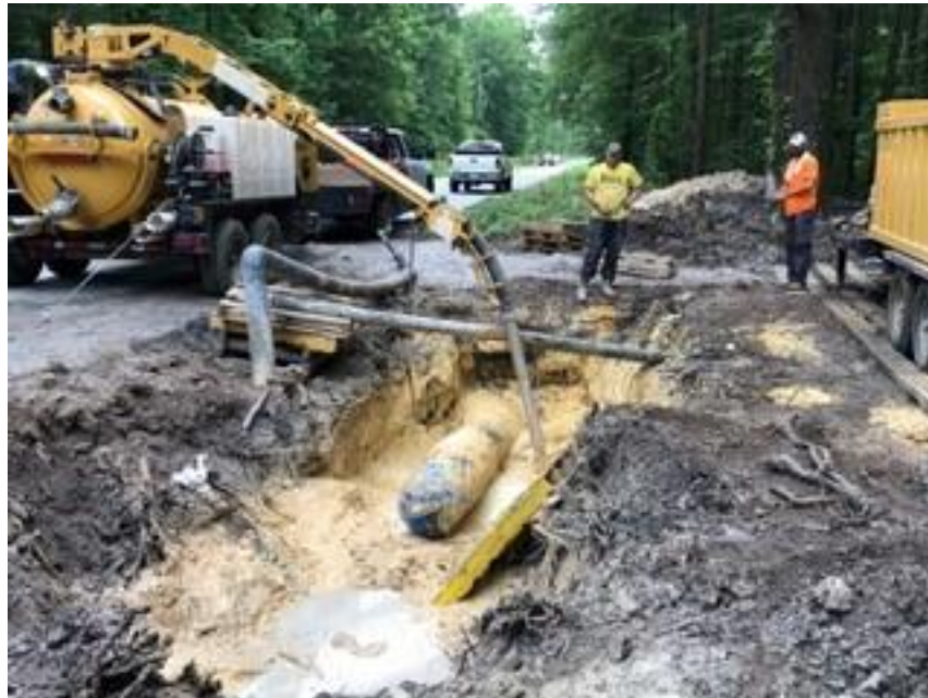
Photo 1: Bore under road
