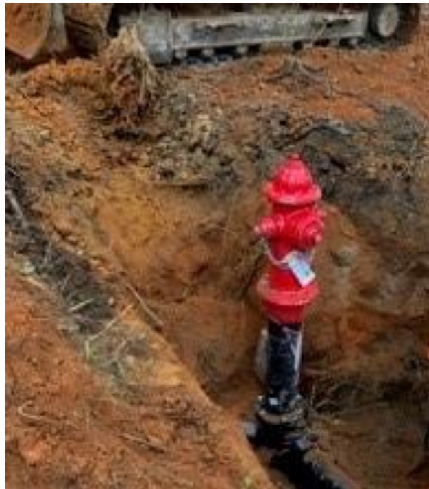
Photo 3: Fire hydrant installation
