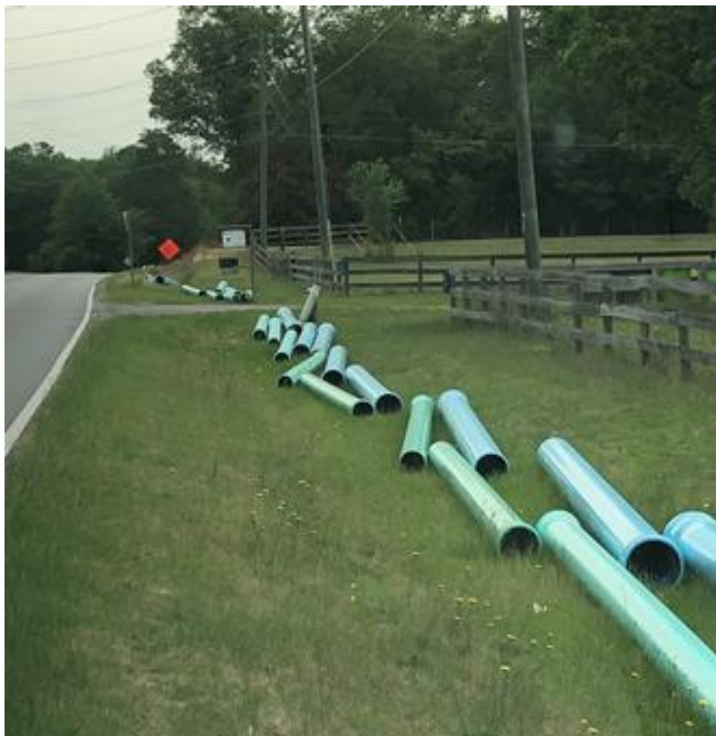
Photo 3: Installing water line on Congaree Church Road.
