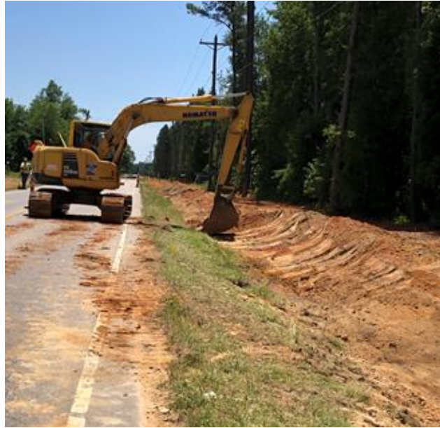
Photo 1: Laying 16” line Lower Richland Blvd
