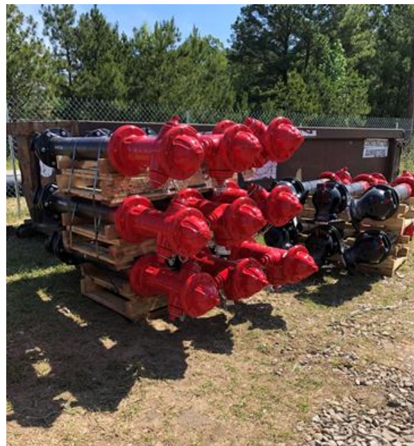
Photo 2: Fire hydrant delivered
