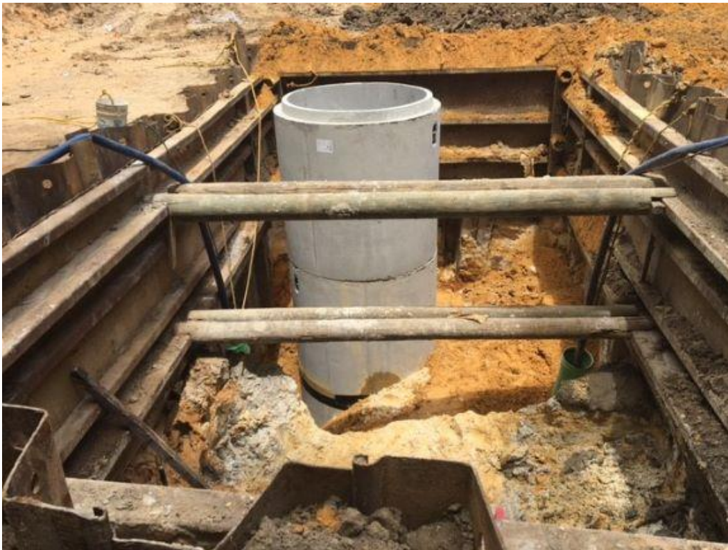
Photo 4: Wet well installed at Hopkins Elementary School.
