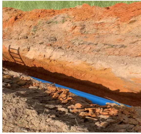
Photo 4: Blue utility pipe
