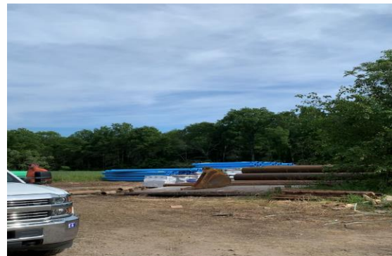
Photo 2: Material Storage Yard
