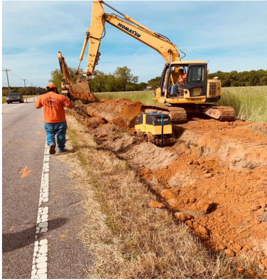
Photo 3: Burying a utility pipe
