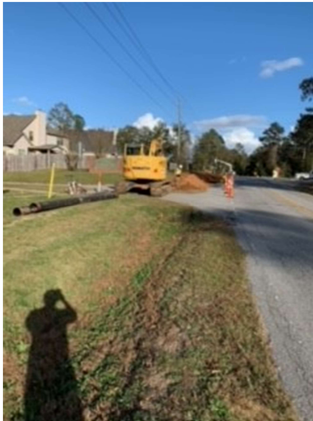
Photo 4: Force main install
