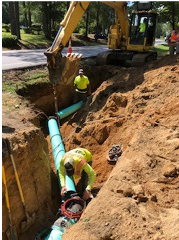
Photo 4: Force main install
