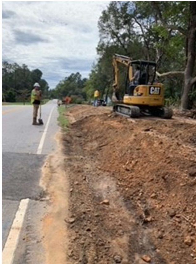
Photo 4: Force main install
