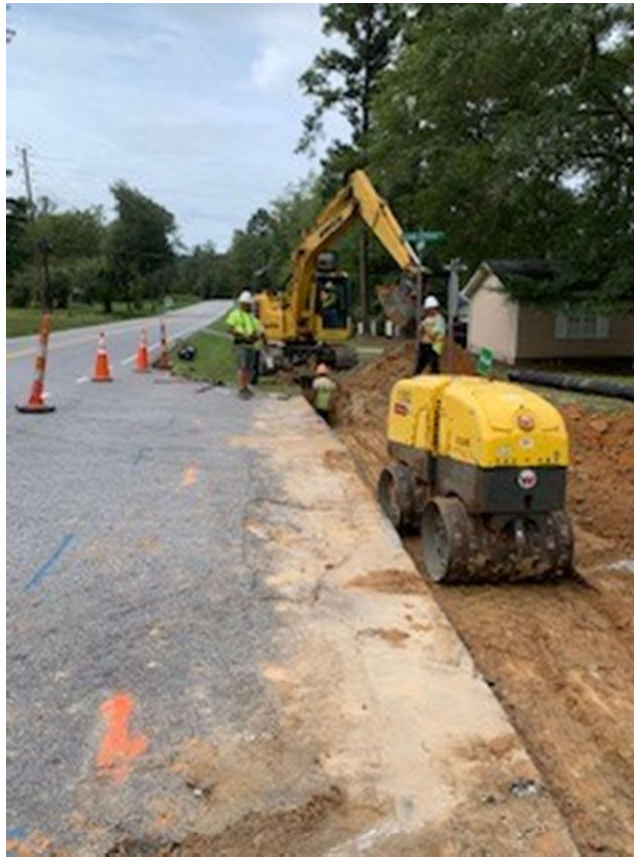
Photo 4: Force main install
