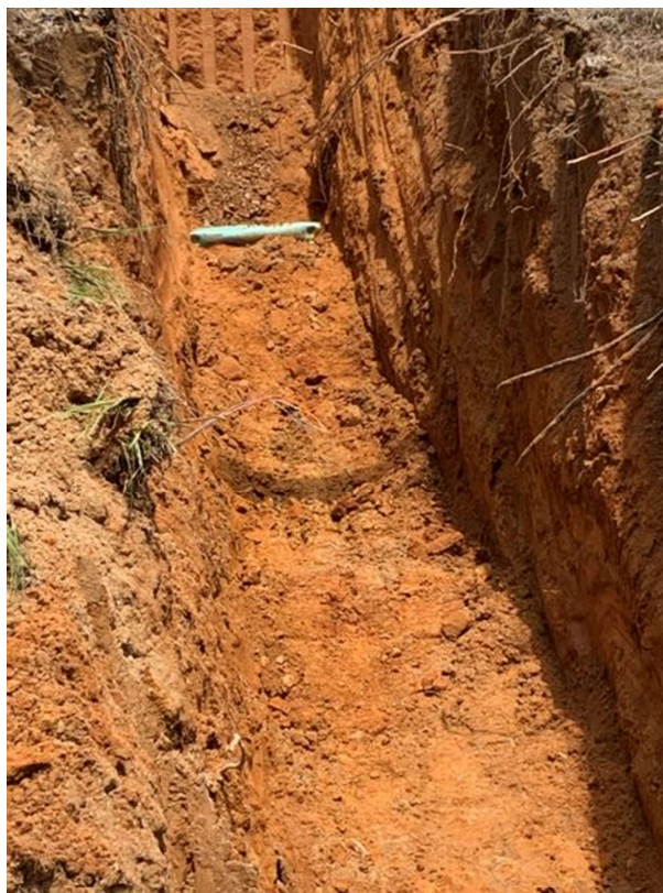
Photo 3: Service connection install
