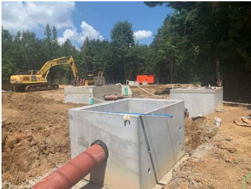
Photo 2: Valve pit install
