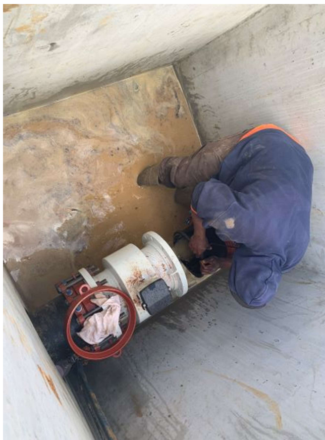
Photo 2: Meter install
