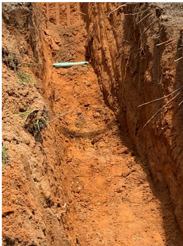
Photo 3: Service connection install
