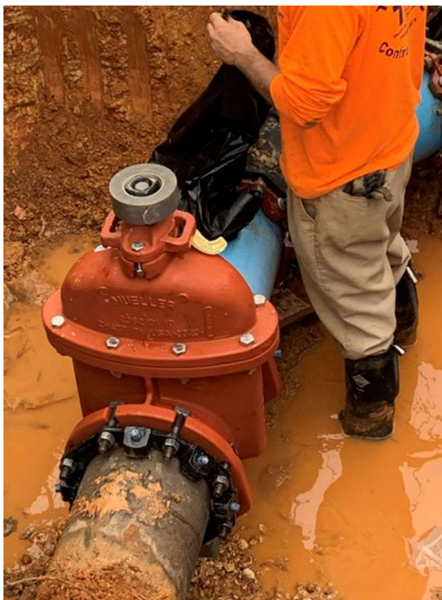
Photo 2: Valve install
