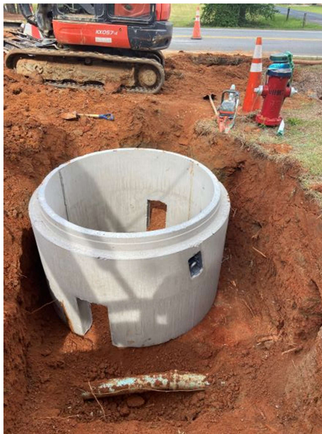
Photo 4: Air release valve install
