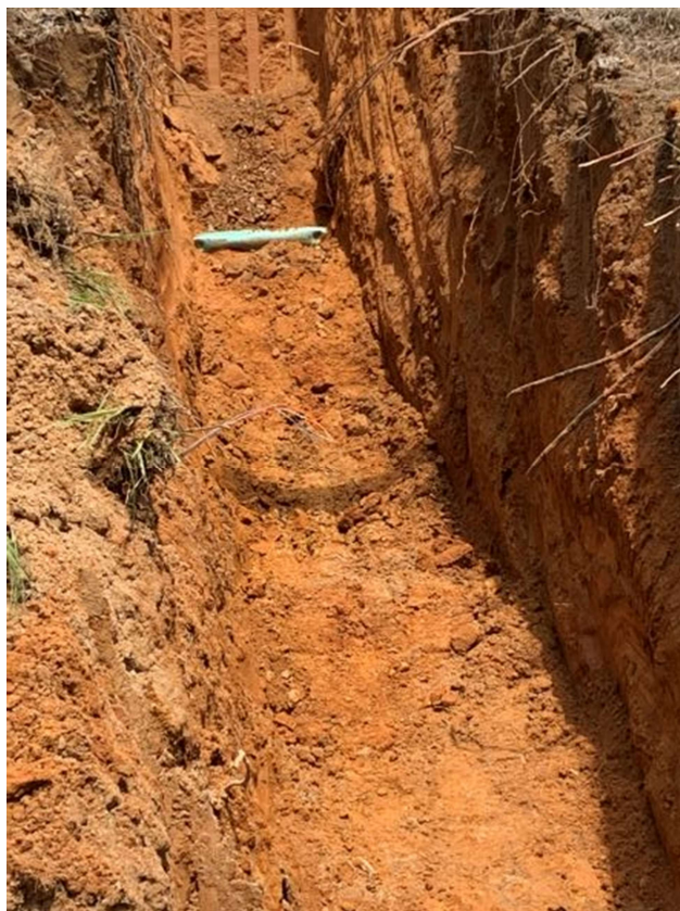
Photo 3: Service connection install
