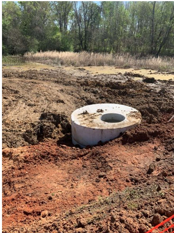
Photo 1: Valve pit install
