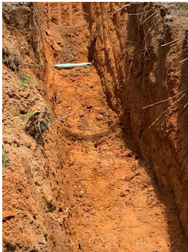
Photo 3: Service connection install
