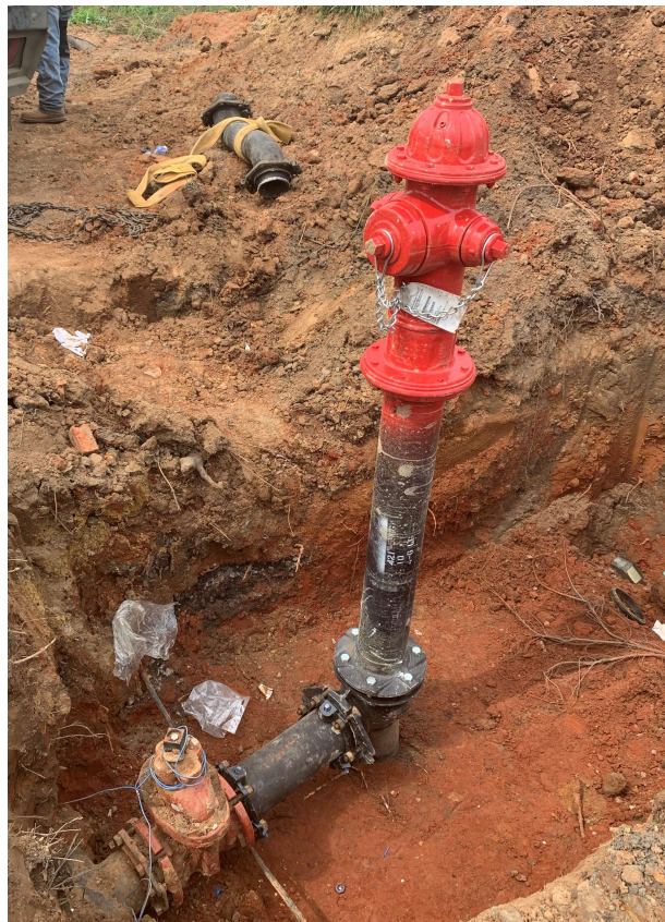
Photo 1: Hydrant install
