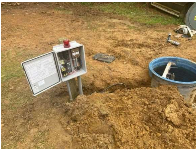
Photo 3: Grinder system install
