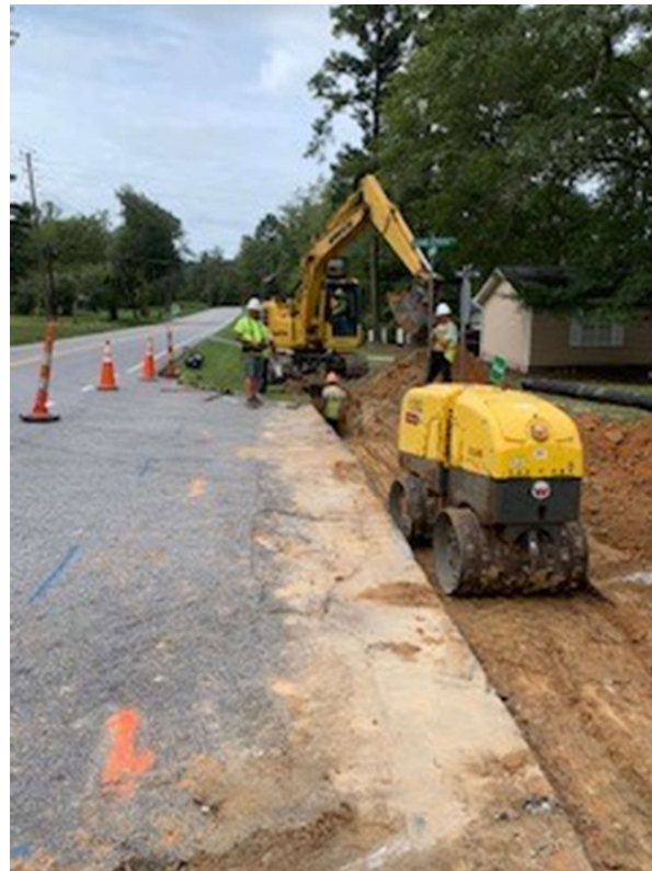
Photo 4: Force main install
