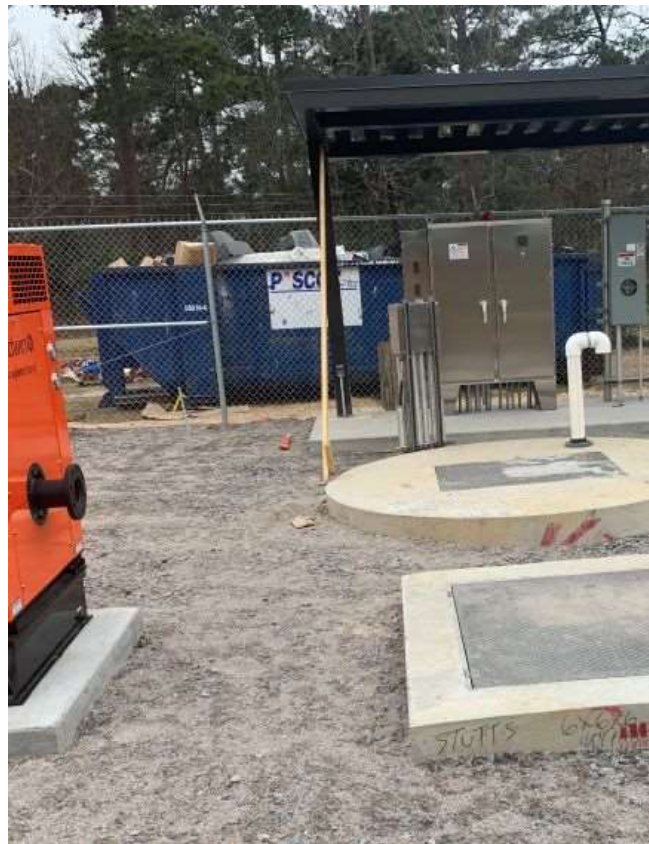
Photo 4: Force main install
