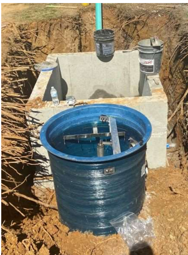
Photo 3: Grinder system install
