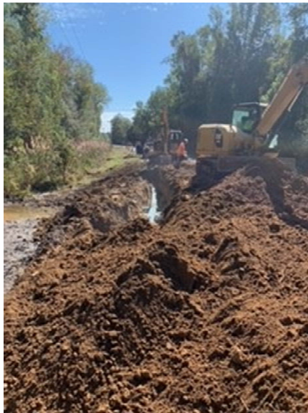
Photo 4: Force main install
