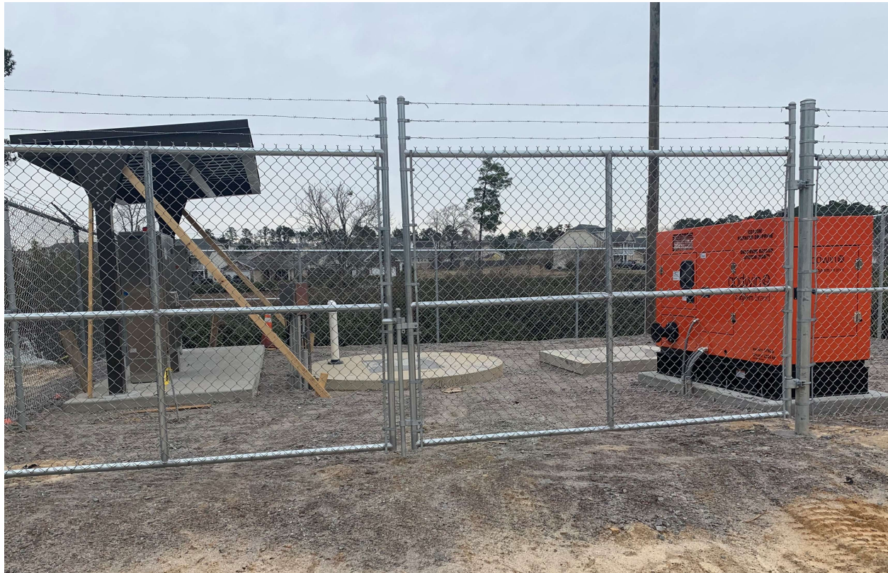
Photo 4: Force main install
